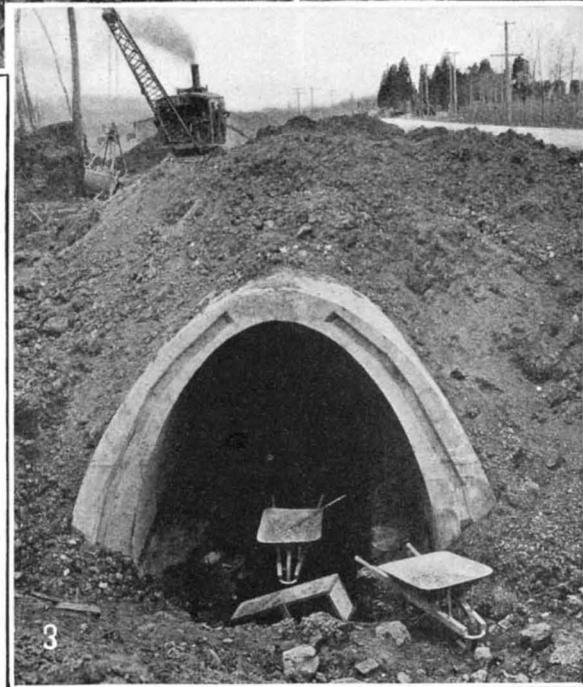
1. The mechanical traveler that moves the forms from section to section after the concrete has hardened. 2. A temporary track inside the conduit carries miniature cars that support the interior metal forms. These forms, too, move forward with the work, pulled by rope cables. 3. Groove in the end of a section, to take the asphaltic joint
