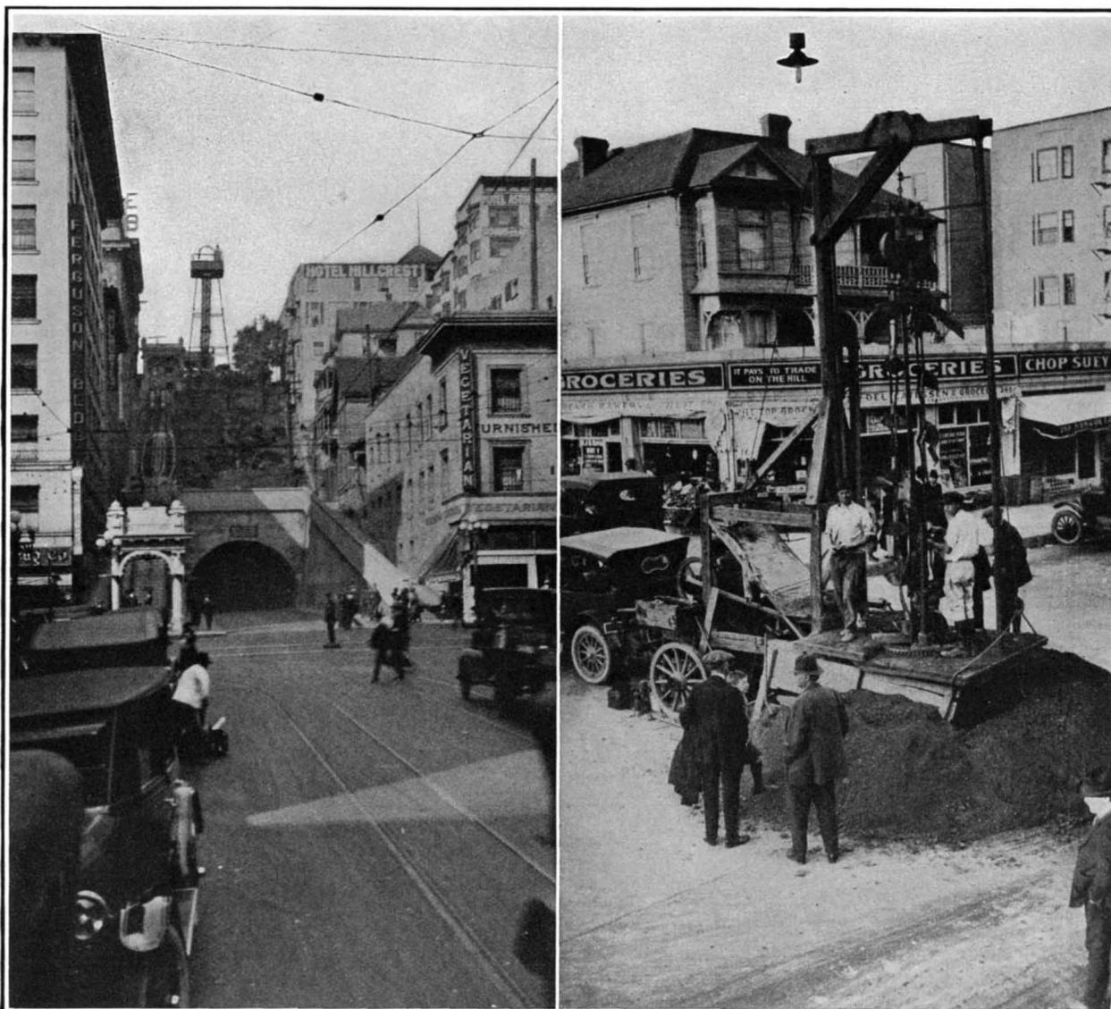
Left: Street view showing east end of the Third Street tunnel, Los Angeles. One of the new ventilating ducts is close to the observation tower. Right: Sinking the 42-inch ventilating shaft, 90 feet deep, with the use of a manhole digger
