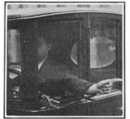
Novel type of window that makes hand signalling from a closed car easy
