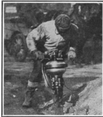
This portable drill carries its own gas engine, and is tied down by no air hose or current connection
