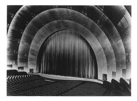
Radio City Music Hall, view of stage, c. 1933. Although the shape of the proscenium suggests expanding waves of sound, the huge arches were actually made of sound-absorbing plaster. Loudspeakers were hidden behind the grilles that were integrated into the arches. Photograph, n.d., Museum of the City of New York, Theater Collection.
