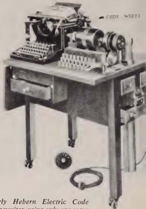
*Early Hebern Electric Code Typewriter*, using only one rotor
