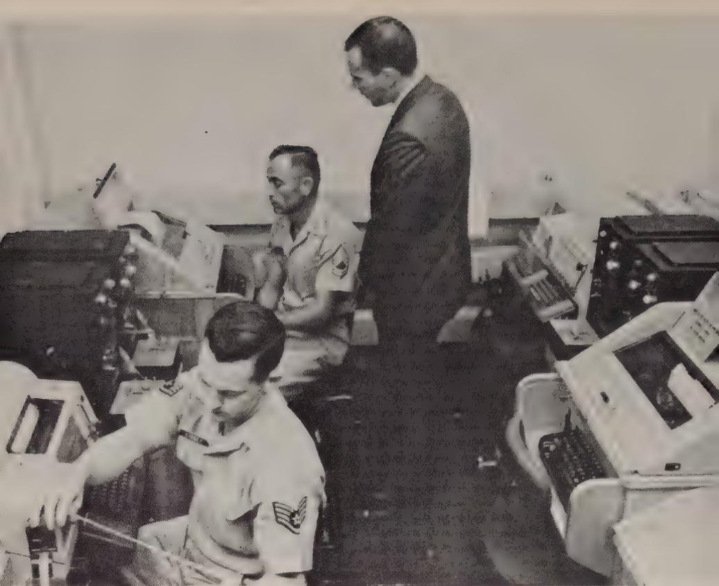
*American end of the Moscow-Washington "hot line," with black one-time tape cipher machines standing between the teleprinters*
