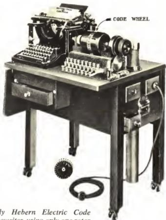
Early Hebern Electric Code Typewriter, using only one rotor
